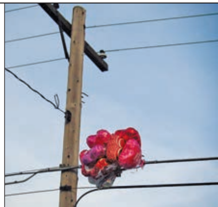
Valentine balloons and power lines are likely to create an unromantic outage.
