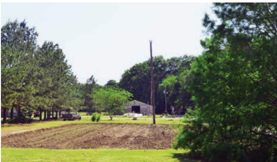
These wires were connected to the pole that was hit by the tractor. Wires were down across the highway stopping traffic until crews arrived.
