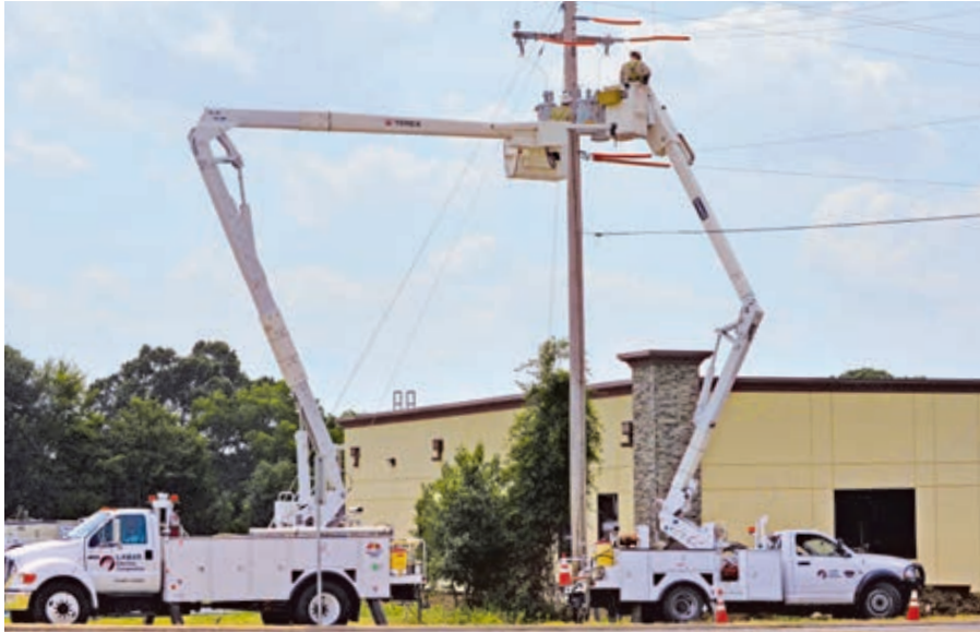
Charles Brazeal and Cory May install transformers to provide power to the new dental office.
