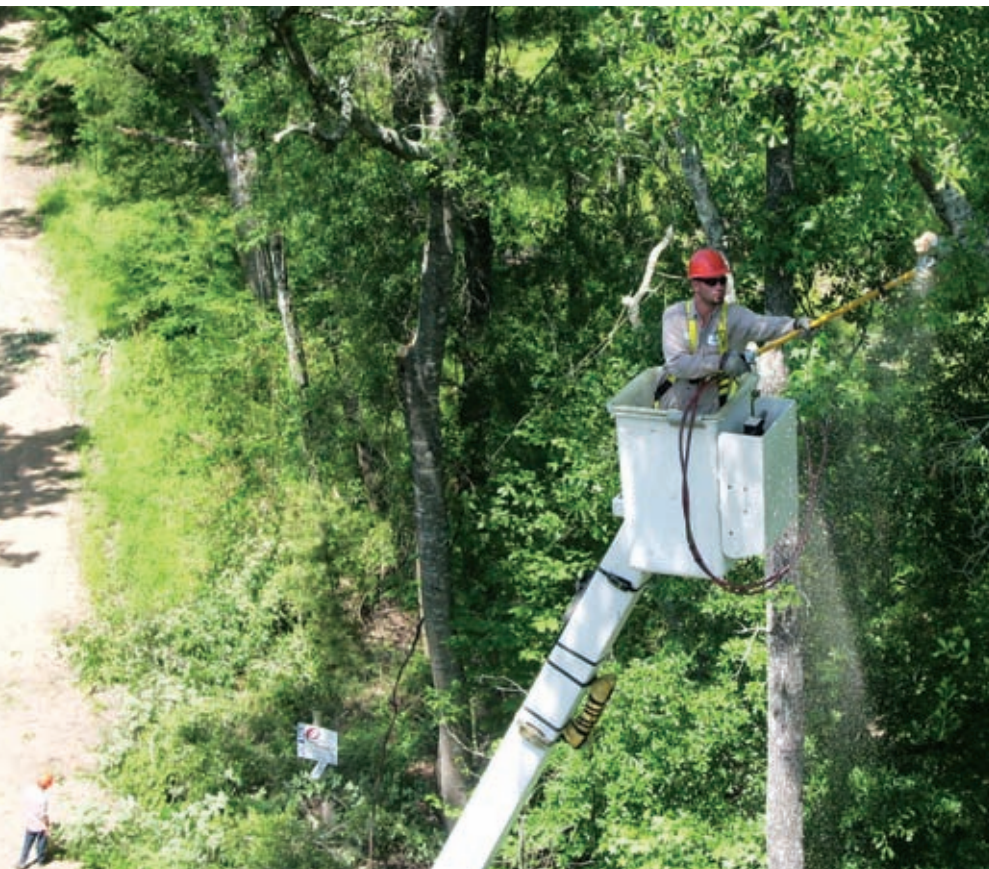
Timely right-of-way clearing improves service reliability and reduces operating costs.
